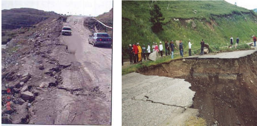
Fig.2. View of the road after landslide.
